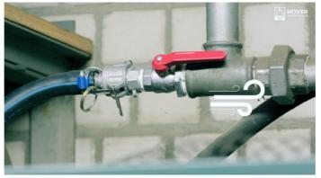
Slowly turn on the air supply to the control unit by turning the red lever.
