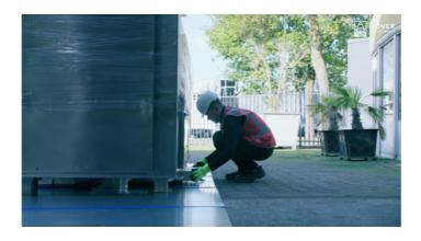
Place the air control unit in the most logical position to perform the movement. Mostly the unit is placed in front of the object in the direction of the movement. Or on one of the sides if that is more practical.
